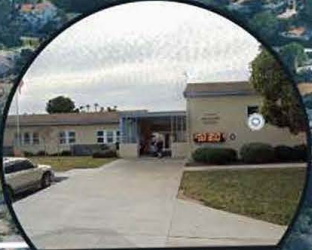
ROSEBANK ELEMENTARY SCHOOL
